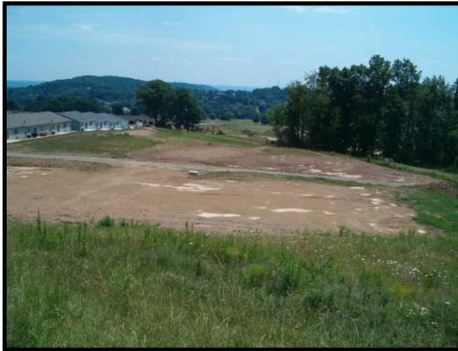
As more land development in the Township occurs in hill ground, there is potential for increases in the velocity of stormwater runoff, and associated problems such as erosion and stream sedimentation.
