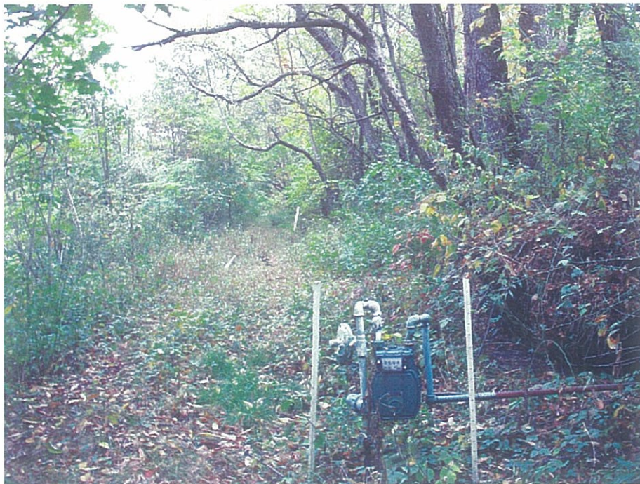
R9-2 Gas meter on gas line bench
