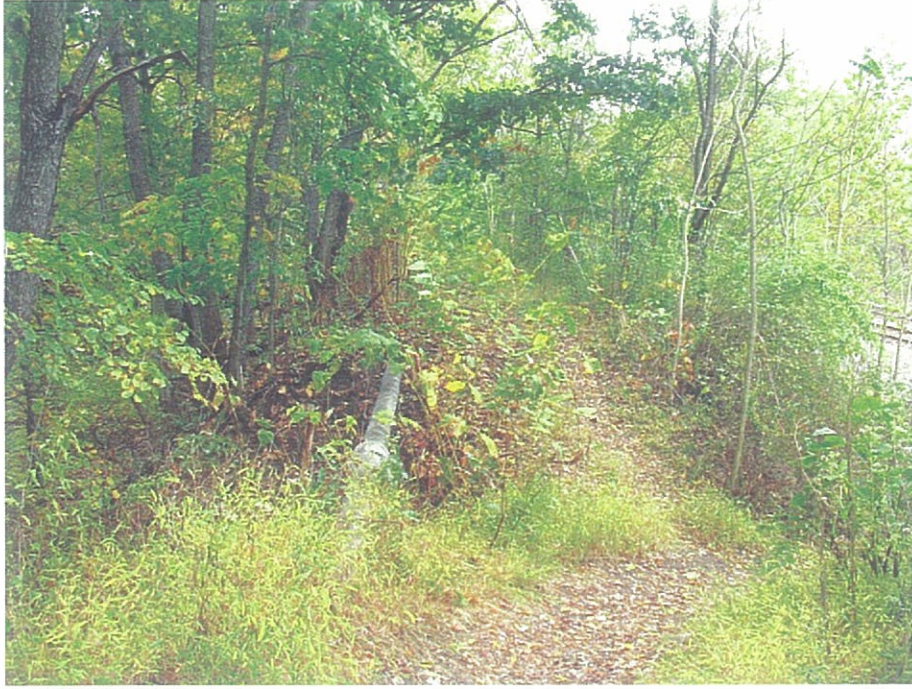
R9-1 Exposed gas line near western end.
