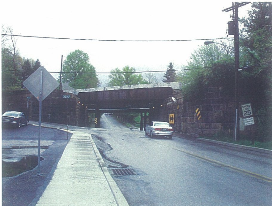
B10-3b Walnut Street RR overpass with low clearance spans removed
