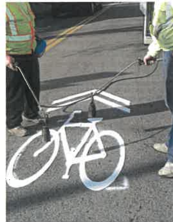
photo credit: BikePGH Sharrows installation: Friendship Avenue, City of Pittsburgh
