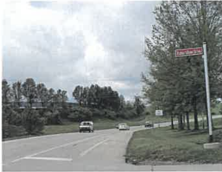
Buffered bike lane: Rose Street, Indiana County
