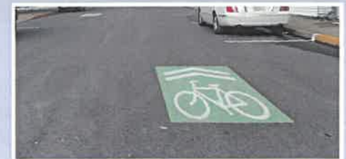
Shared lane markings in green boxes, also known as green sharrows: 8th Street, Indiana, Indiana County
