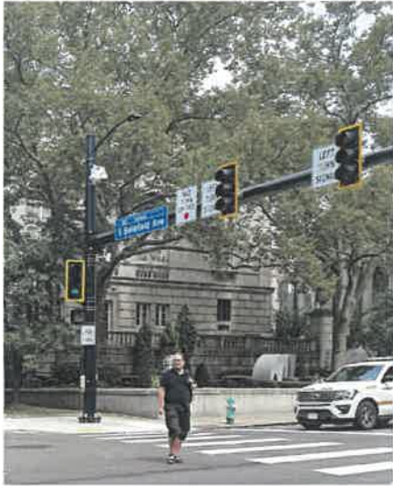
Bicycle signal: Forbes and Bellefield Avenues, City of Pittsburgh
